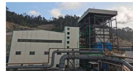
PT.DSI 1*150MW 发电厂
