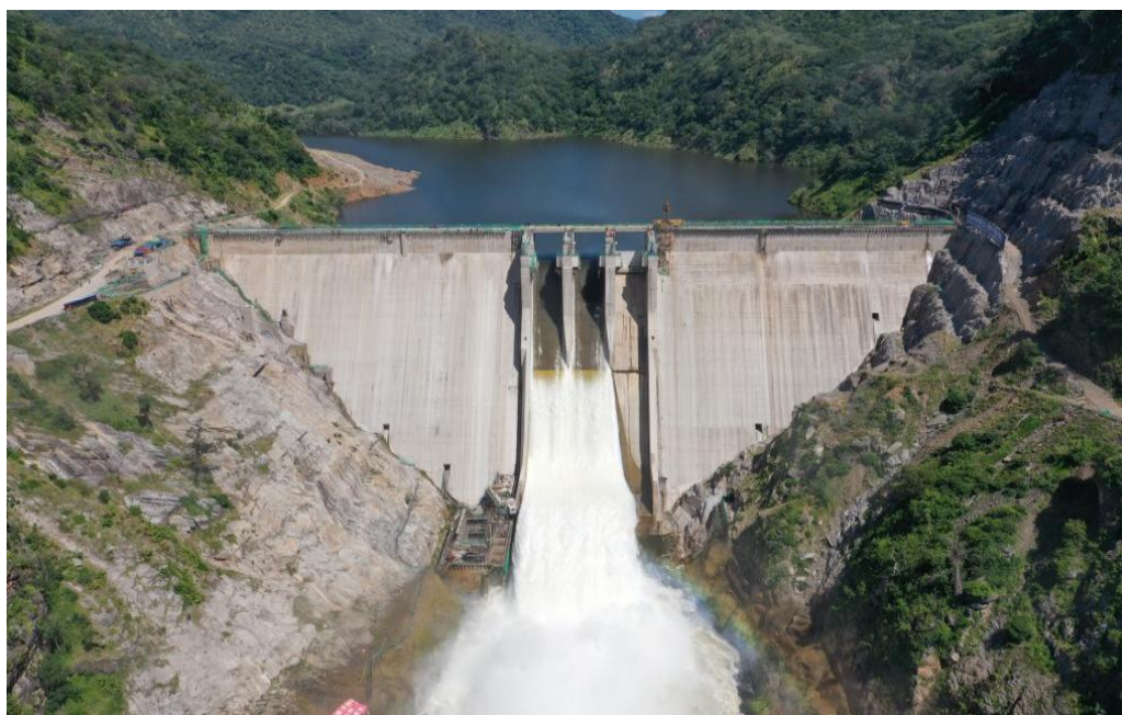
凯富峡水电站大坝
